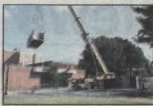
HVAC Unit Installed on Willett Gym Roof Pg. 2
