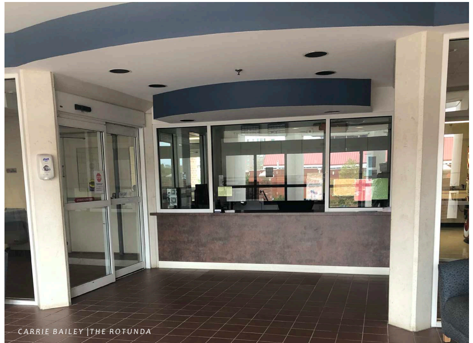
Along with Curry, Arc Hall is closed due to maintenance.
