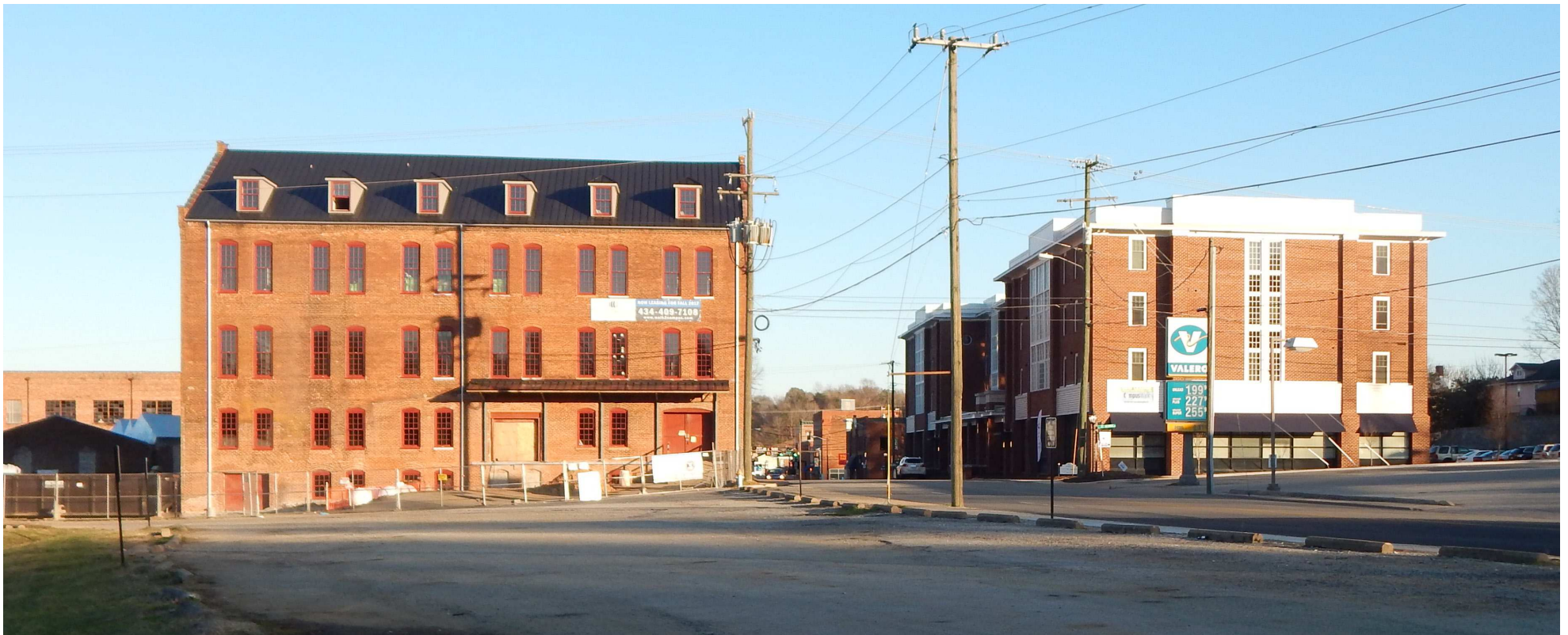
Walk2Campus apartments is currently renovating buildings along West Third Street, constructing new, luxury apartments targeting college residents.
