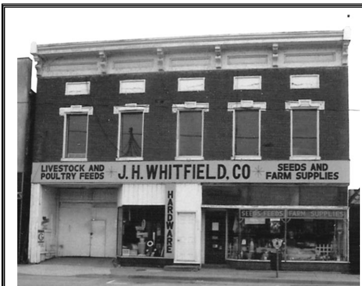
The Whitfield Building, constructed in the early 1860's, is the oldest storefront building still in its original form in Farmville. The building was designed from noted architect Asher Benjamin's early 19 th century books on architecture. Of interest is the Greek Key over the windows on the second floor.
