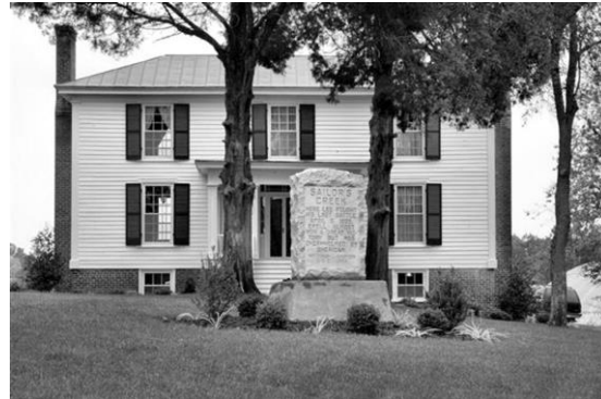
Lockett House now
