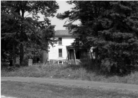
Lockett House before
